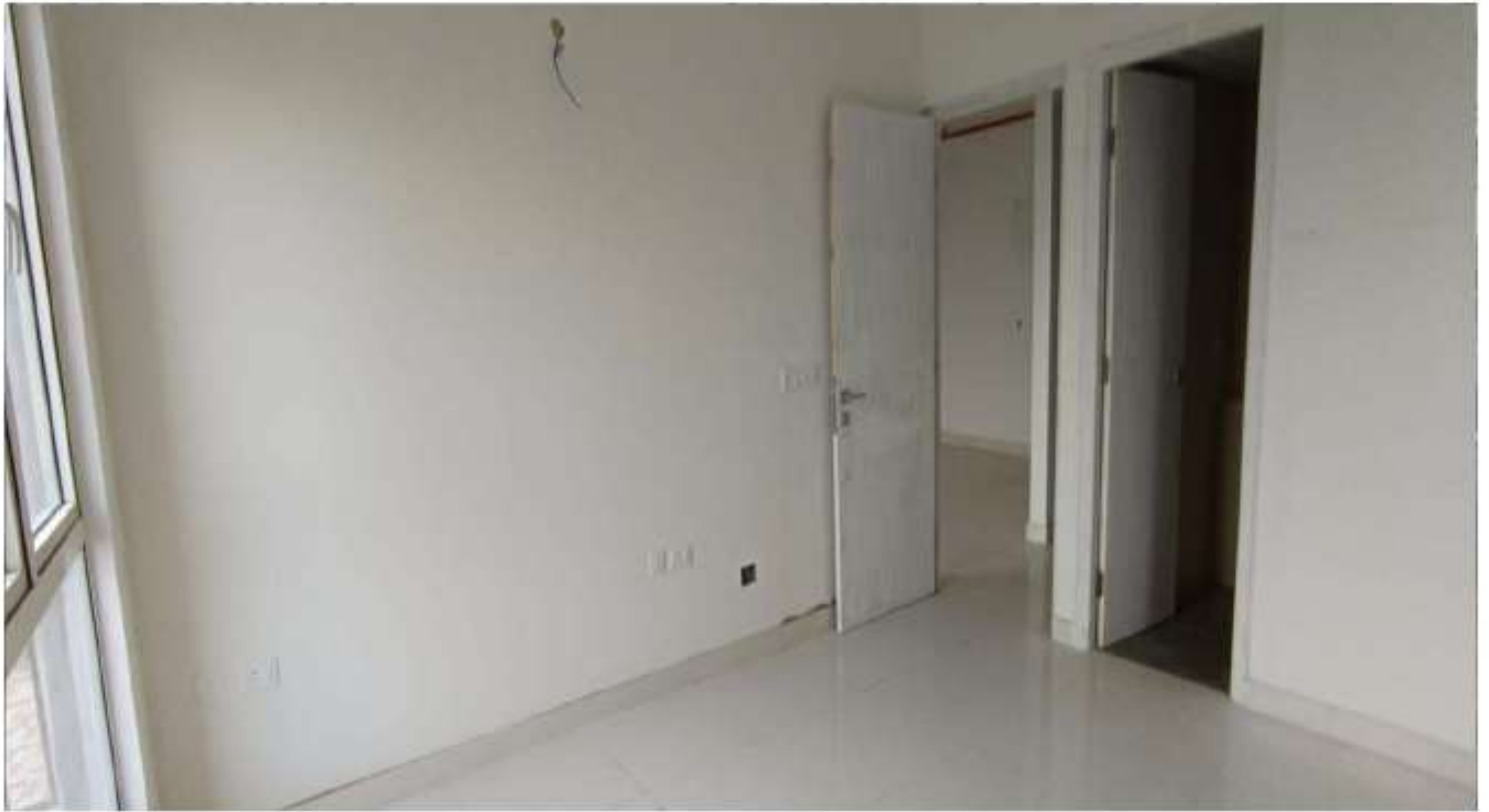
BLOCK 2 & 3 FLOORING COMPLETED
